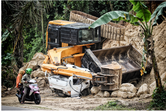
Figure 1.5: A crawler excavator collapsed, as it was operated on unstable ground [113, CC0 1.0].
